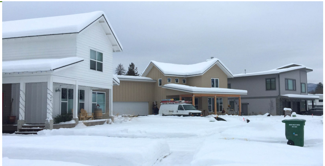
High Point on Second Street has seen a number of new single family homes built after the Final Plat was approved in 2017
